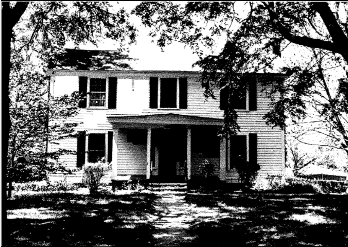
Figure 1. The historical front façade and porch of the, then called, “Ball House” in c.1985 (photo from the Pictoria History of Roswell )
