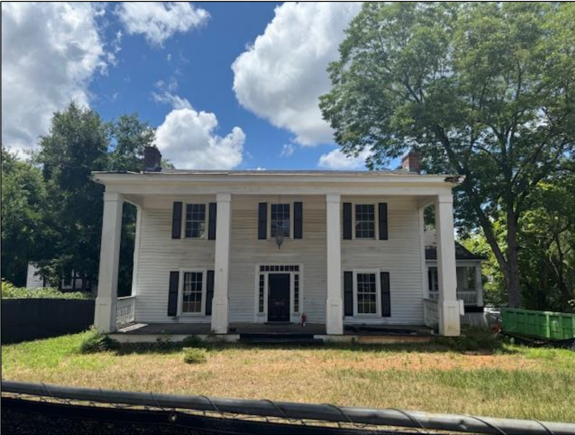
Figure 2. The existing front façade of Founder's Hall/1076 Canton Street (photo from Staff)
